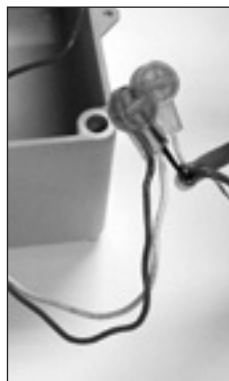
Figure 11.12 - Splice wire
