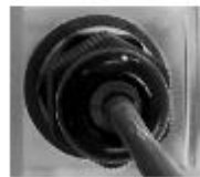
Cable Gland with cable
