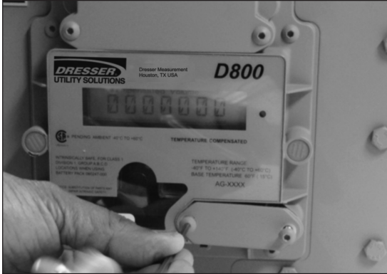
Figure 9.1 Example - Remove two button head screws
