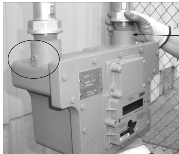
Figure 11.1 Example - Differential pressure taps are located on the inlet and outlet connectors
