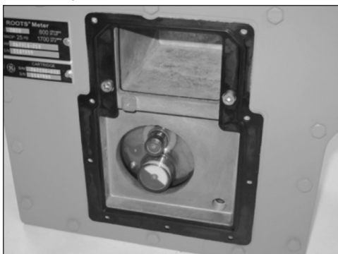
Figure 9.13 Example - Place gasket onto meter
