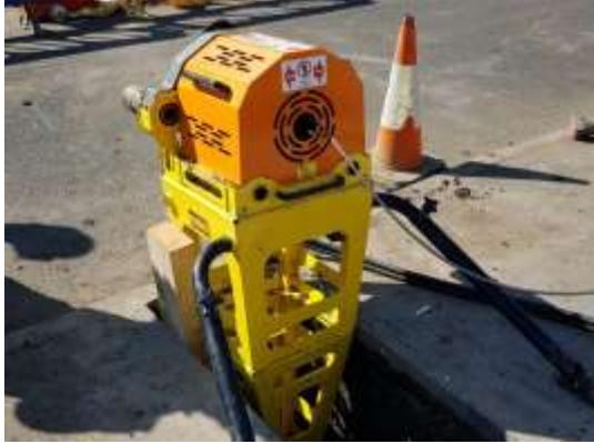
The system utilises a specially constructed steel pulling cable assembled with our patented pulling ferrule. The single use cable is inserted through the pipe being replaced; the pulling ferrule is engaged onto one end of the pipe and the other end of the cable is wound onto the spool of the Pipe Puller.
