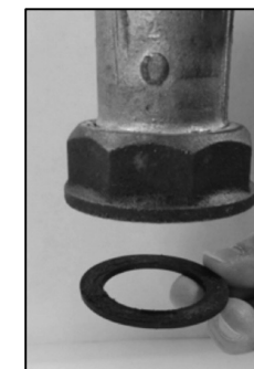
Figure 5: Proper installation of washer into swivel
