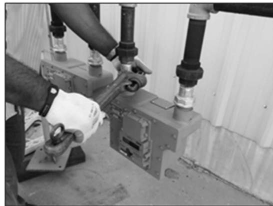
Figure 9: Use a pipe wrench to tighten swivel nuts
