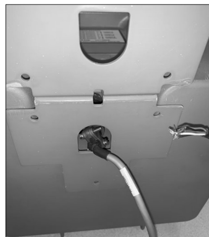
Figure 24: Properly positioned mounting bracket
