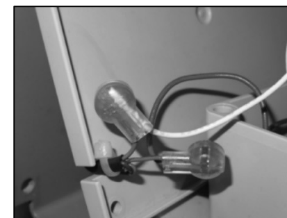
Figure 27: ERT cable properly routed through the back plate
