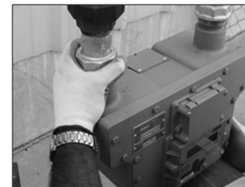
Figure 6: Connect meter ferrule into swivel nut on the gas supply side
