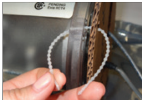
Figure 8.15 -Remove cardboard cover
