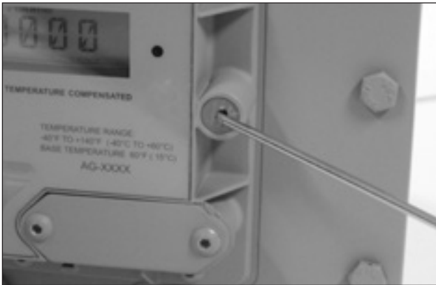
Figure 9.6 - Retirez les joints
