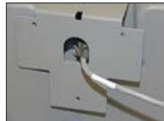
Figure 7.18 Example - Pull cable through the center hole
