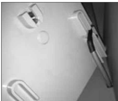
Figure 7.22 Example - Meter cable routed across back plate
