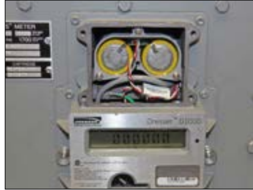
Figure 9.30 Example - Battery pack in place
