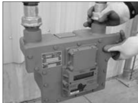
Figure 7.3 Example - Connect meter outlet to swivel nut on the downstream side
