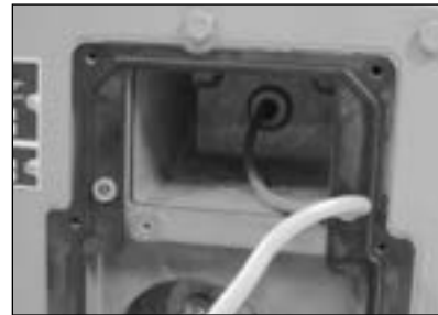
Figure 9.15 Example - Run cable through back of meter
