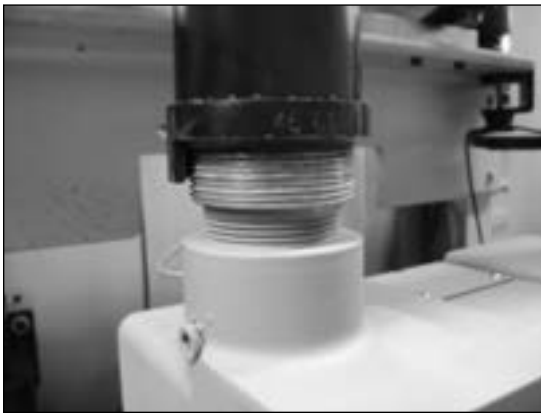
Figure 10.10 Example - SNAP connections properly fitted to meter
