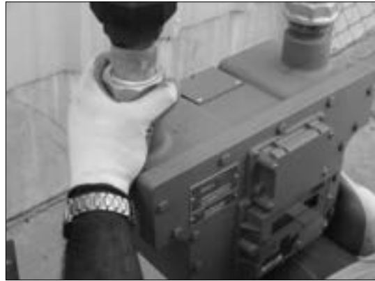
Figure 7.2 Example - Connect meter ferrule into swivel nut on the gas supply side
