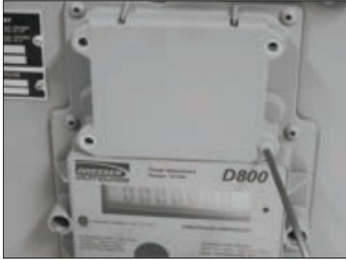
Figure 9.27 Example - Remove 4 screws on battery cover
