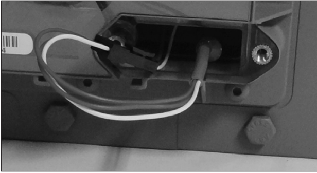
Figure 9.23 Example - Push temperature probe into probe well
