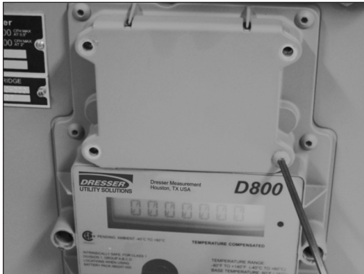
Figure 9.7 Example - Remove 4 screws on battery compartment
