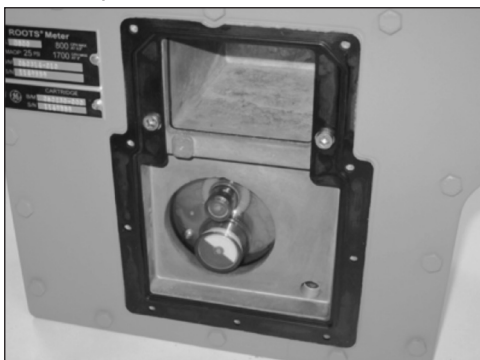
Figure 9.13 Example - Place gasket onto meter
