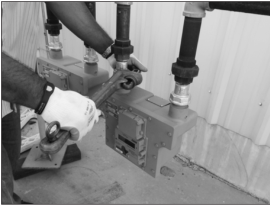
Figure 7.5 Example - Use a pipe wrench to tighten swivel nuts
