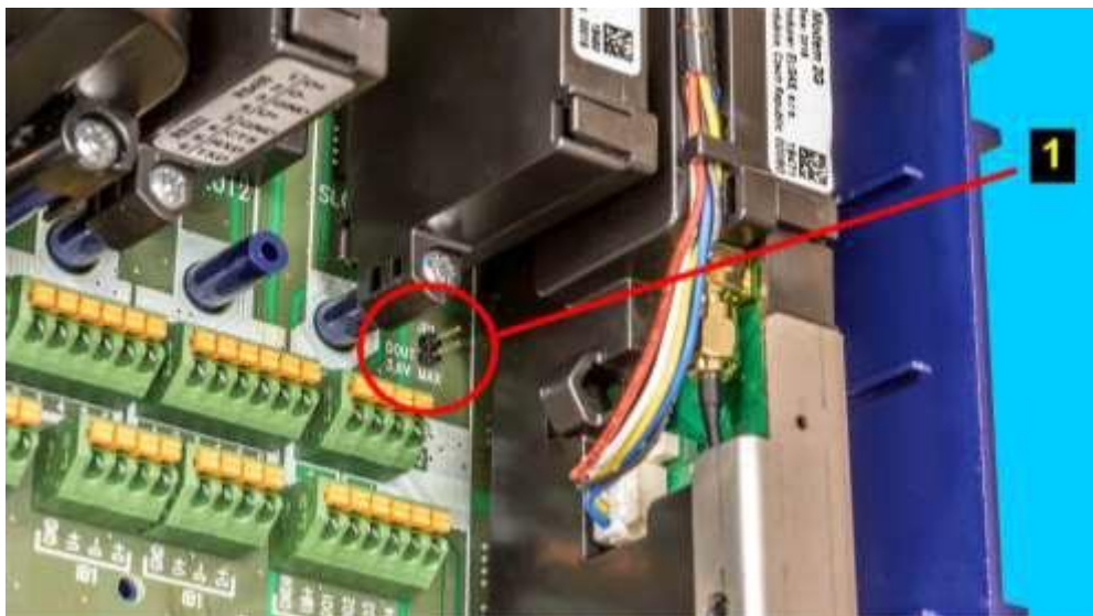
Fig. 42 Placing JP1 Jumper on I/O Board
