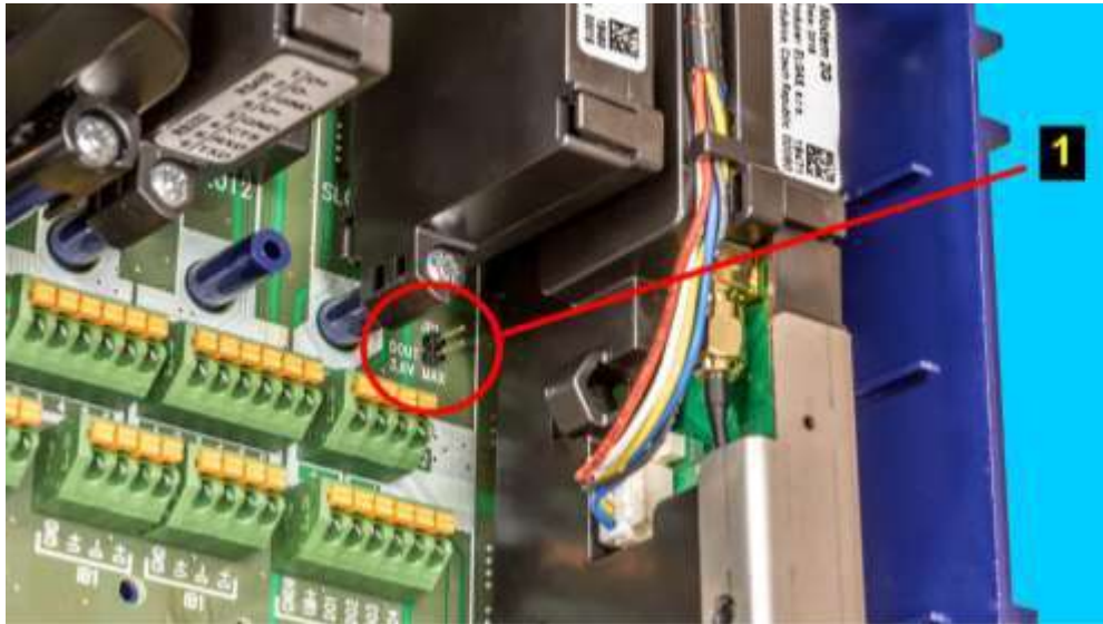
Fig. 42 Placing JP1 Jumper on I/O Board
